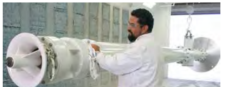
NSF certified epoxy coating being applied to pump
